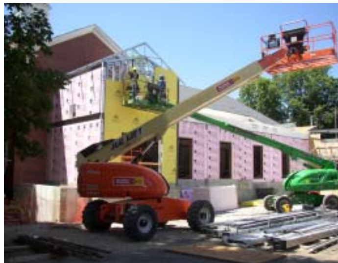
Exterior of new ramp connecting the Gathering Space to the sanctuary
