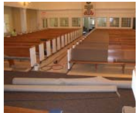
Carpeting and upholstery work in progress . . .
