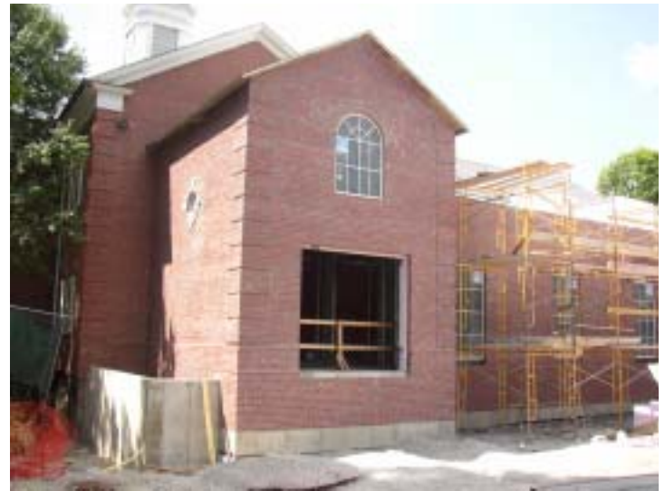
Photos show the extension on the east side of the church, the scaffolding for completing the brickwork and the opening for the door leading to the south parking area.
