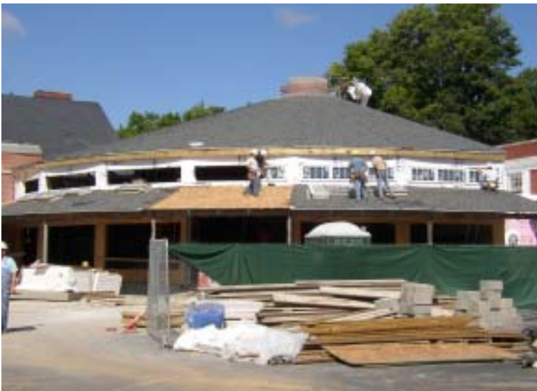
Photos of the Gathering Place as workman shingle the roof and view of the Gathering Place clerestory windows, which help reduce or eliminate the need to use electrical lighting during the day.
