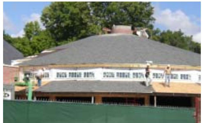
Photos of the Gathering Place as workman shingle the roof and view of the Gathering Place clerestory windows, which help reduce or eliminate the need to use electrical lighting during the day.
